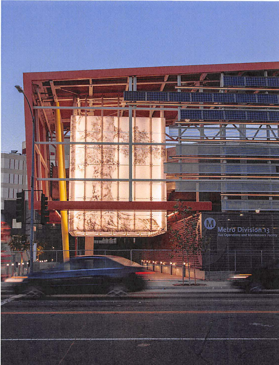
Detail, Division 13 Bus Operations and Maintenance Facility, El Aliso de Los Angeles , Christine Ulke, Artist.
