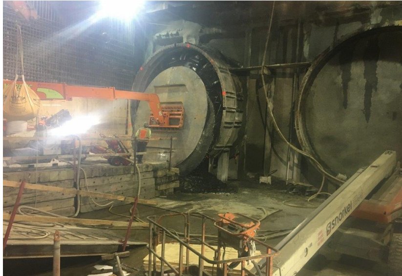
C1045 200404 135PM Fairfax Station View of STS' E. Hammerhead T.B.M. break through, N. tunnel. Looking NE
