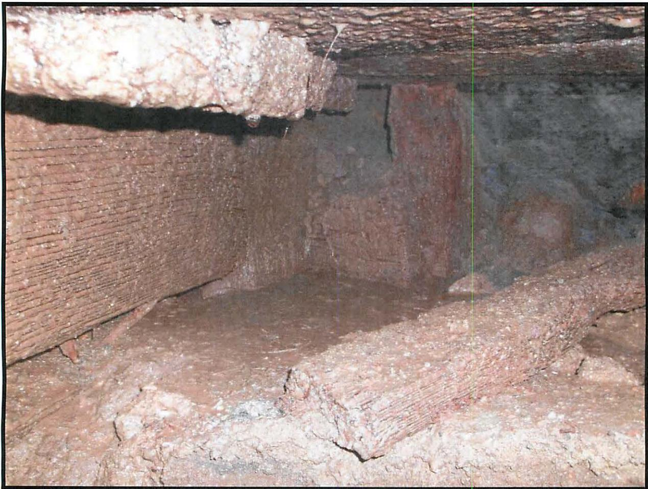
**The voids consisted of a set of streetcar tracks overlying a subterranean wooden engineering structure apparently made to raise the tracks on their approach to the Macy Street Viaduct.**
