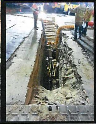
**Sandy soils required trench to be exposed and backfilled with slurry in order to stabilize the trench path.**
