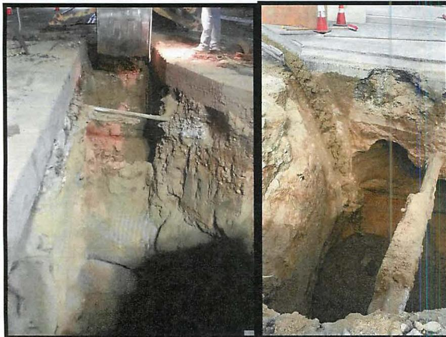
**Underground obstructions including unknown and unused utility infrastructure limited mechanical equipment within the trench.**
