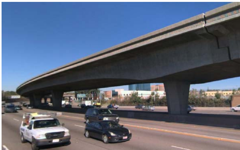
I-5 Highway Viaduct – Santa Ana
